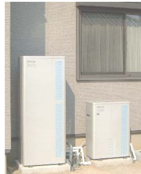
Japan: Large-Scale Demonstration Project for Stationary PEFC system Stationary 1kW-class PEFC CHP systems for residential throughout Japan
