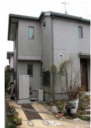
Japan: Large-Scale Demo Project for Stationary PEFC system – over 2000 units installed
